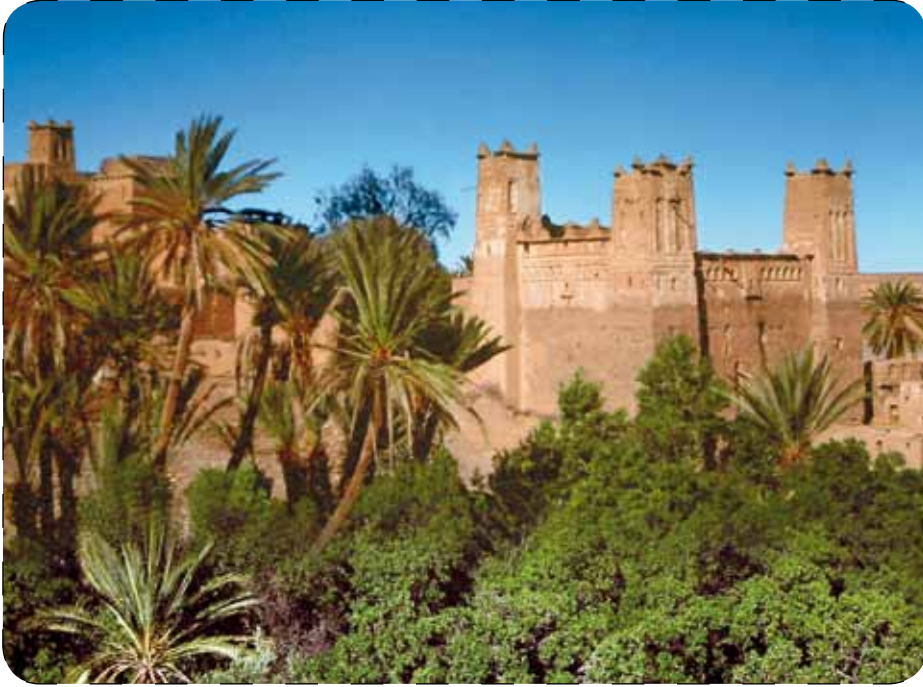
Kasbah in Morocco made of raw earth: "viable" city
