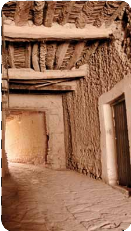
Roads still in use and well maintained
