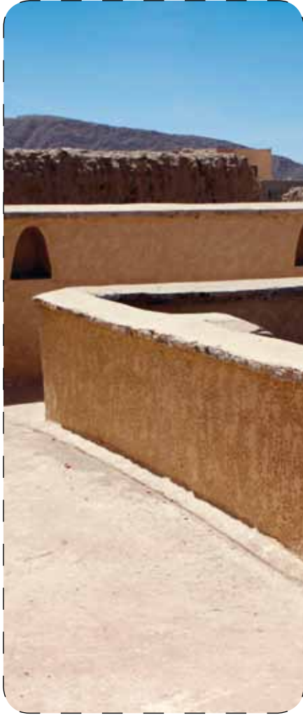
Figui, restored terrace
