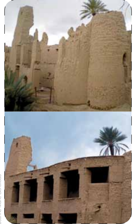
The wall of the Ajdir plaza, before and after restoration
