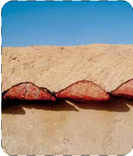
Cover detail, redone according to tradition
