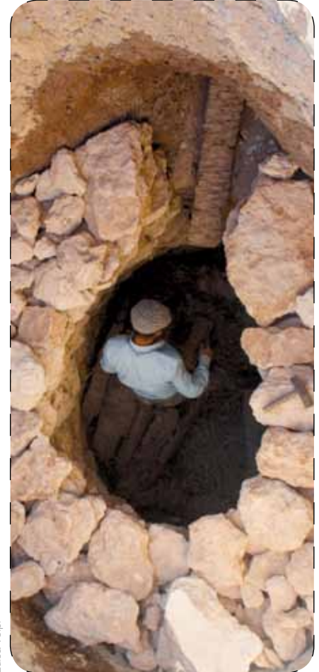
Preparation of lime kiln before burning (protection of walls)
