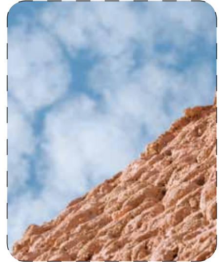
Old structures deteriorating
