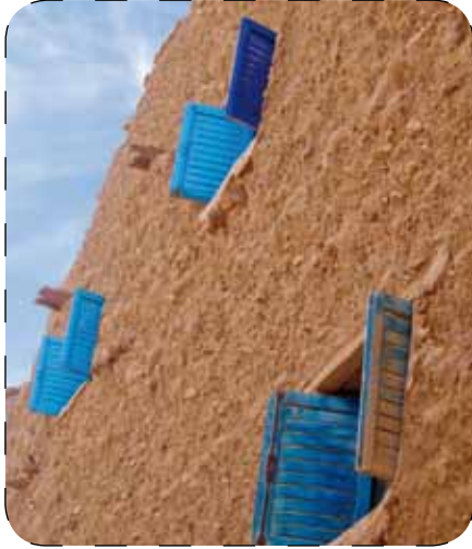
Building being restored in Figuig
