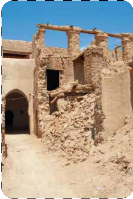
Restoration and ruins in Figuiç
