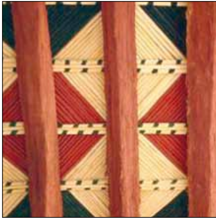
Type B floor (beams and oleander rods)
