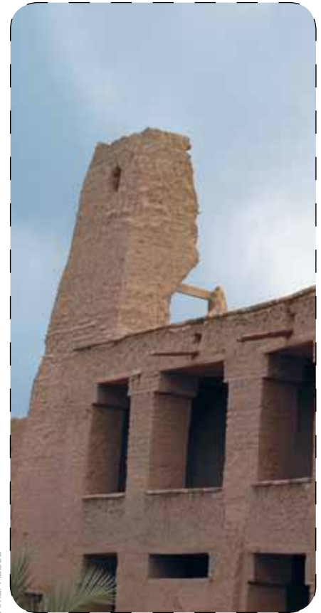
Ongoing restoration of the Ajdir Wall
