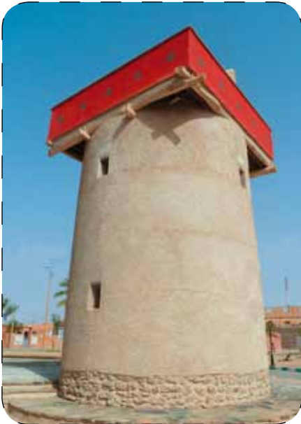
Tower for infokiosk made of raw earth by the NGO Africa '70
