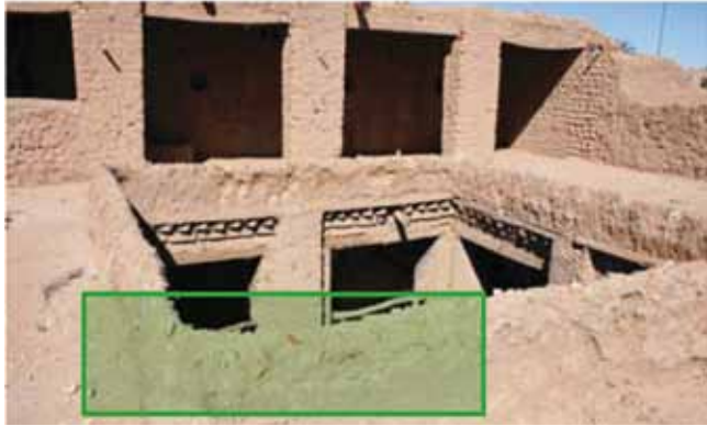
Progression of erosion of the entire constructed system
