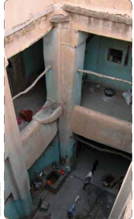
Courtyard and gallery of Figuig homes
