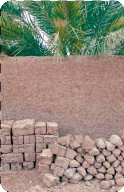
Molded blocks and adobe made of mud
