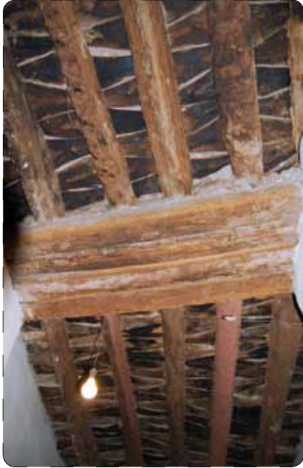
Old floor maintained and unaltered
