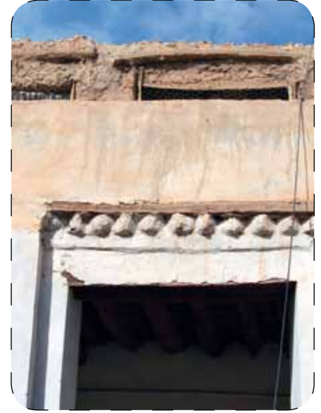
Zoom in on an architrave made of palm wood
